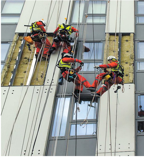
Removal of previous ACMPE panels
