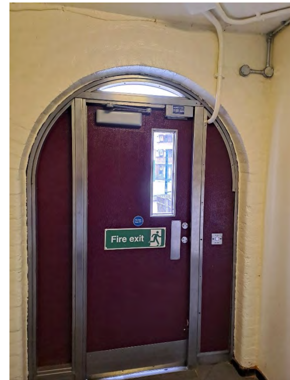
Main exit fire door at 1-19 Aborfield.
