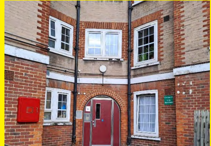
External Emergency lighting at 1-19 Aborfield.
