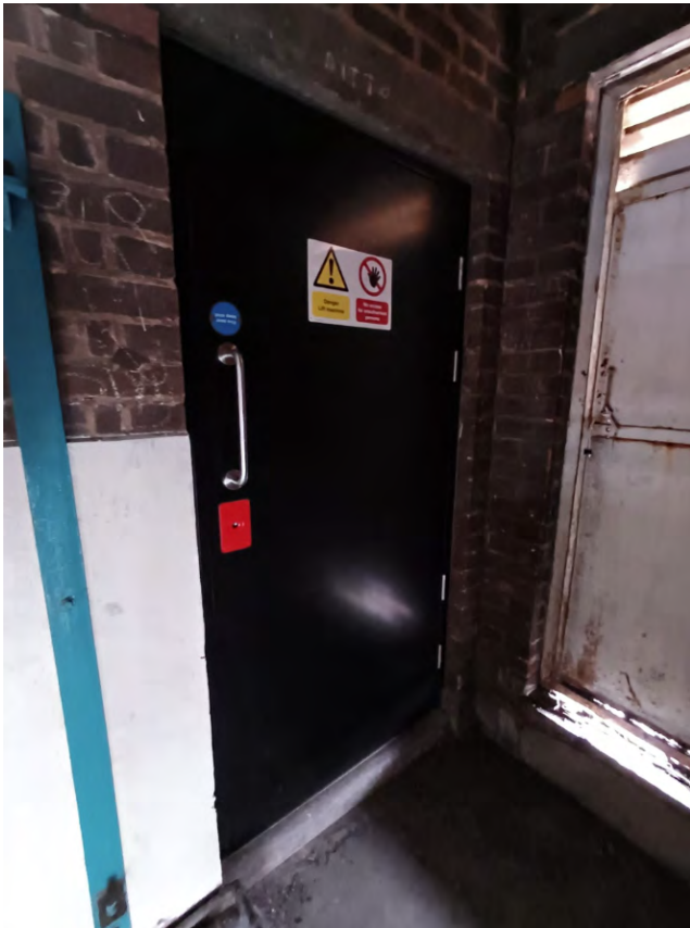
Lift Motor Room Fire Door at 1-19 Peperfield.
