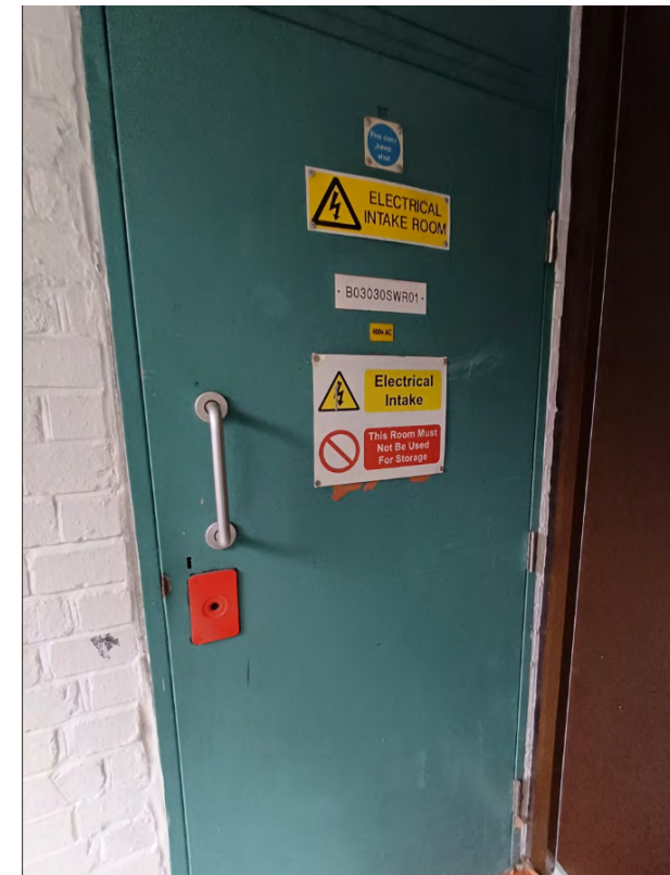
Electrical Intake Room Fire Door at Peperfield.
