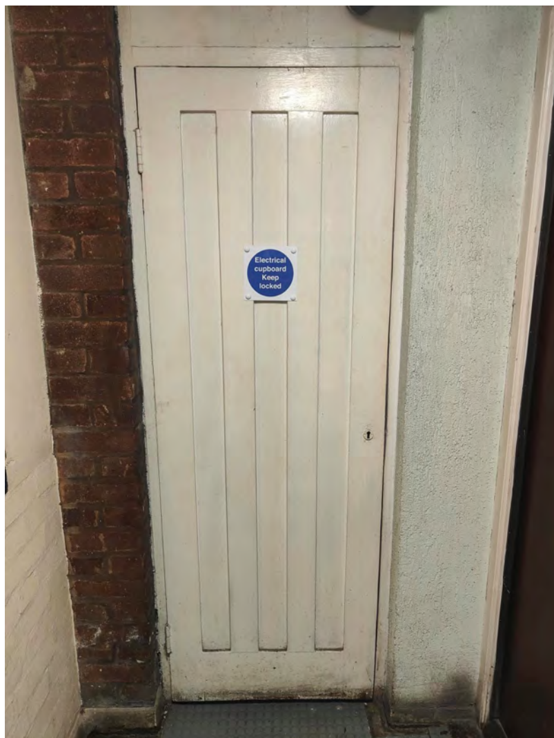
Electrical intake cupboard fire door at Fleetfield.
