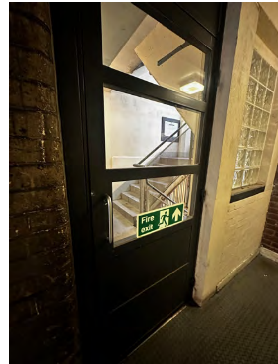
Communal Fire Door at 1-25 Fleetway.
