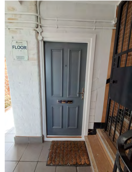
Front Entrance Door at 1-32 Mead Close.
