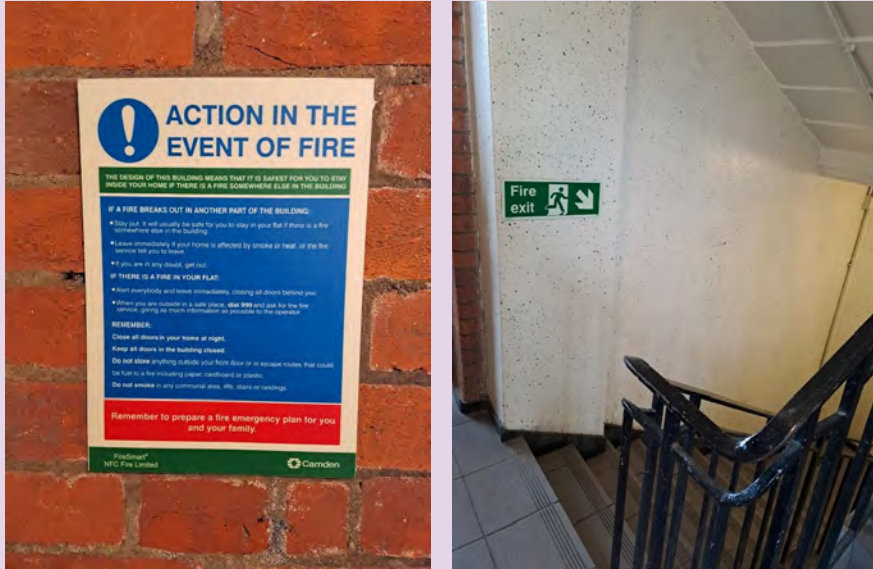
External Fire Action Notice and a Fire Exit Sign at Greatfield House.
