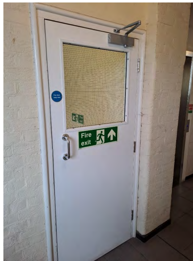
Internal fire door on escape route at Greatfield House.
