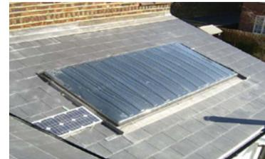
A solar water heating system collects thermal energy from the sun via roof-mounted panels and uses the energy to pre-heat the domestic hot water supply, thus reducing heat demand from the boiler. With a conventional gas-fired central heating system a dual-coil hot water cylinder is used:
