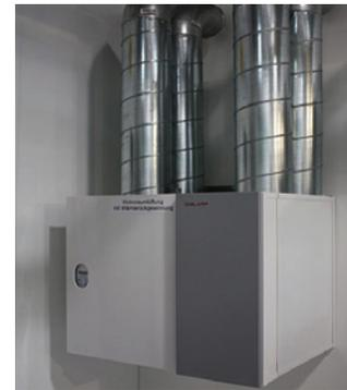
In properties with good air tightness, a continuously operating ventilation system may be required. This can either be a single fan with ducts to the 'wet' rooms and the kitchen (centralised mechanical extract ventilation), or several fans running continuously (decentralised mechanical extract ventilation). Both types of systems can benefit from low power fans, to reduce the electricity use. Fresh air is supplied by trickle ventilators that may be humidistat controlled.
