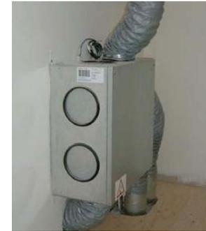
Whole house MVHR systems run continuously, extracting moist stale air from kitchens and bathrooms and supplying fresh air to living spaces and bedrooms, via ducts. The systems recover some of the heat from the extracted air and use it to pre-heat the incoming fresh air. Modern MVHR systems use energy efficient DC fan motors for low fan power, and incorporate plastic cross-flow heat exchangers to achieve heat recovery efficiencies as high as 90%.
