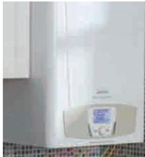
Domestic CHP replaces a conventional gas-fired central heating boiler and generates electricity (2kW or less) as a by product of providing heat and hot water.
