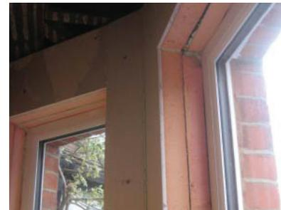
Insulation is fixed to the inside of the wall, and then covered by a plasterboard lining. The installation must also include a vapour barrier and/or air-tightness membrane; sometimes a ventilated space (on the cold side of the insulation) and a wiring void (on the warm side of the insulation and air barrier) are also included.
