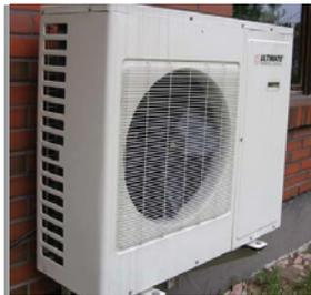
A heat pump works by extracting heat from an external source and supplying it to the property for heating or domestic hot water. Heat can be extracted from the ground, from water or from the air.
