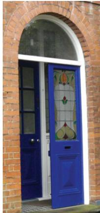
Heat is also lost through external doors and this can be reduced by thermally upgrading your existing external doors, replacing them with more efficient modern doors or adding a draught lobby inside the front door. These measures do not require planning permission.
