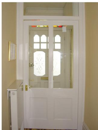
A draught lobby can make a small improvement in the thermal performance of a house by reducing heat loss through the front door and reducing the exchange of warm internal air with cold external air when people enter or leave the house.
